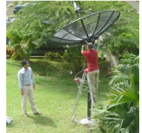
CATHALAC/SERVIR Antenna Installation
